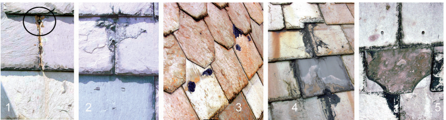
Figure 10: Bad repairs can be found on almost any old slate roof. Some constitute “hidden leaks,” such as #1 above, where a nail has been driven into the top of the slot, caulked, then the caulk has worn off leaving an almost invisible hole in the roof. A bib flashing would have prevented this problem and will still solve the problem if inserted at this time. #2 illustrates the same problem, this time with roof cement rather than caulk. #3 shows “face nails” that have been tarred over — these are guaranteed leaks. #4 illustrates two obvious errors: wrong type of replacement slate and exposed roof cement. #5 is another example of a multiple error — face nails, wrong type of slate and wrong shape of slate. All of the above can be removed and the roof properly repaired.
