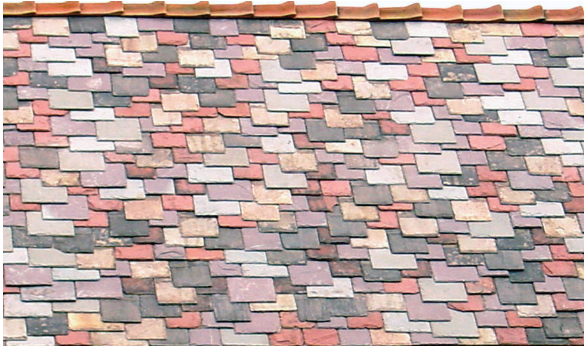
Figure 3: This new slate roof, installed by the author, shows a variety of slate types, including salvaged New York red, Vermont unfading green (the lightest ones), new Vermont sea green (the medium gray ones), salvaged Vermont sea green (the tan ones), Vermont unfading purple (solid purple) and mottled green and purple (purple with green spots, flecks or streaks), Virginia black (the dark gray ones), and Vermont salvaged, polluted sea green slate (the dark ones with the light spots, darkened by air pollution over a century).
