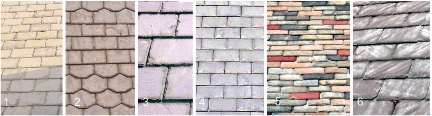
Figure 9: All slate is not the same. The above sampling of slate roofs includes, 1) a 70-year-old Vermont unfading green slate; 2) 110-year-old Pennsylvania black slate (a harder variety); 3) 90-year-old Vermont purple slate; 4) 100-year-old Buckingham, Virginia slate; 5) a mix of sea green slate (also known as semi-weathering green), Buckingham, and NY red slate; 6) Chapman (PA) slate with its characteristic diagonal striations. To see more examples of slate roofs, or to help determine their expected longevities, go to slateroofcentral.com and click on “how to identify your roof.”
