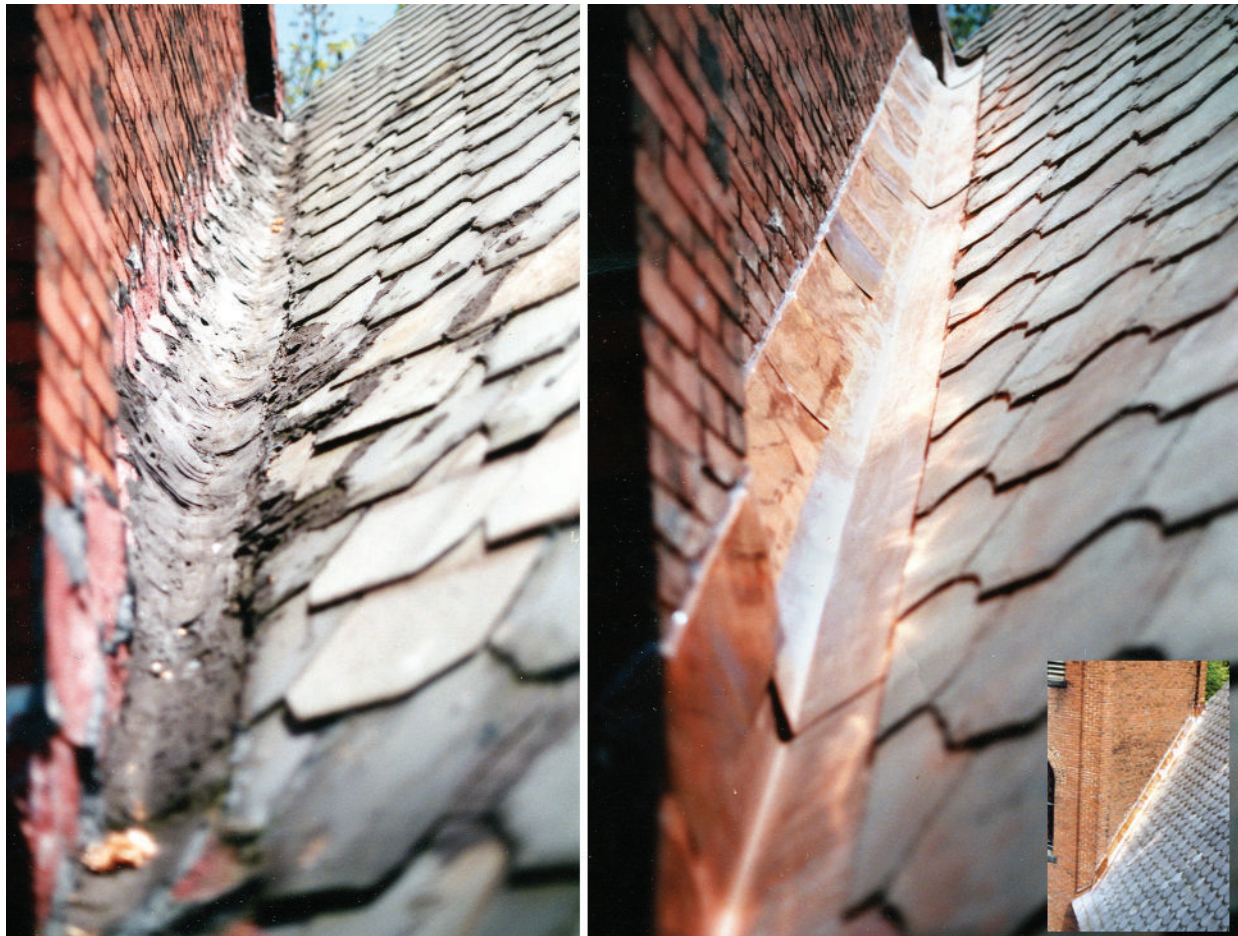
Figure 4: This bell tower on a church built in the late 1800s displays the typical deteriorated flashing and poor maintenance common on slate roofs in the United States today. However, one slater with a helper removed the tarred mess and replaced it with new copper and matching slates in a single work day. Such revitalization of old slate roofs is routine work for experienced slate roofing professionals.
