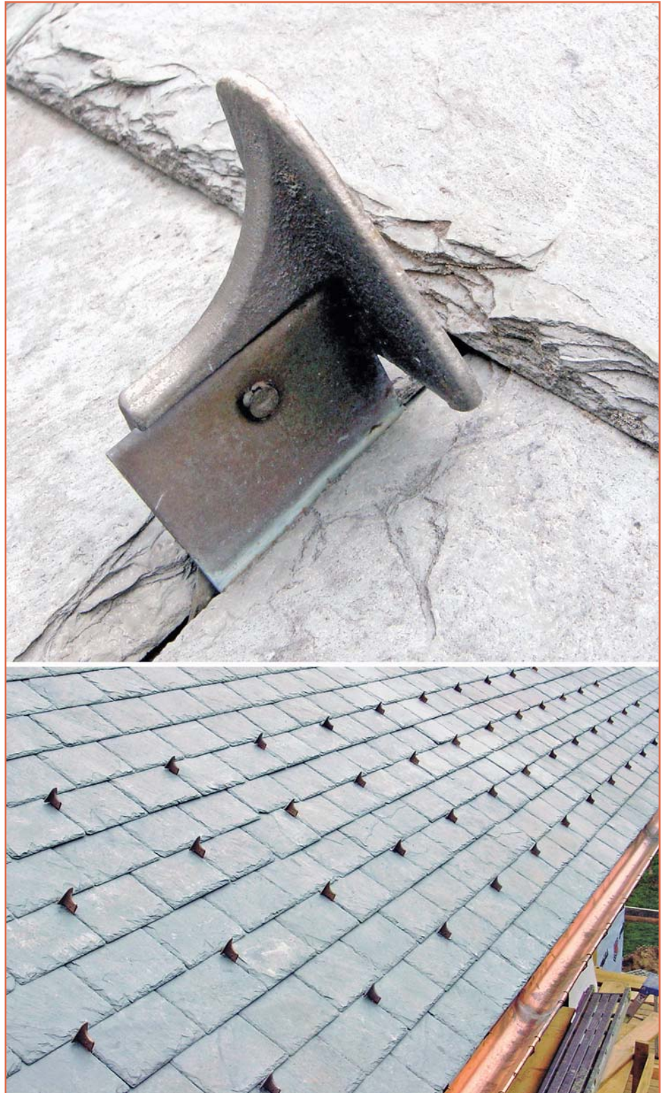
Figure 1 – Mullane's classic 100 and 200 series of snow guards are made from cast bronze and copper. They're available in both standard and retrofit models.
