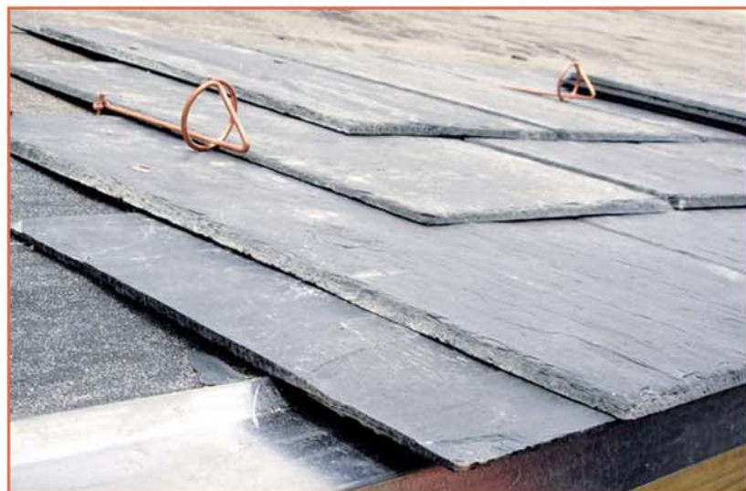
Figure 5 – Copper “loop-the-loop” snow guards are perhaps the least expensive of all snow retention systems. They're easy to install and effective when used in sufficient quantities.
