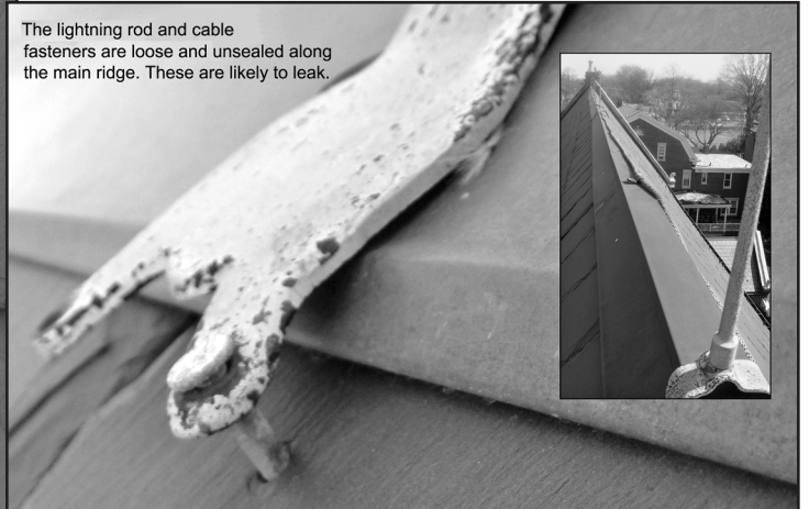
Figure 2 – Exposed, loose fasteners are common sources of leakage. (Photo by Joseph Jenkins.)
