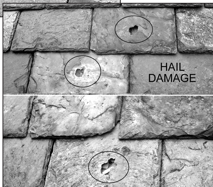
Figure 16 - External punctures, such as from large hailstones, leave holes with sharp edges as shown here. The crater is always opposite the impact side (photo by Joseph Jenkins).
