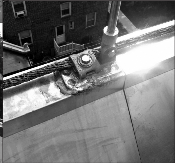
Figure 5 – The leaking lightning protection system was removed and reinstalled by soldering new bronze rod brackets to the new copper ridge, leaving no penetrations through the copper and nothing to leak. (Photo by Chris Short.)
